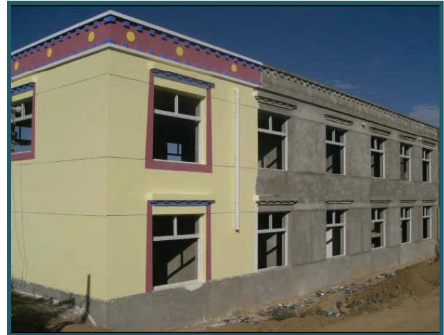
Construction of the Birth Center
